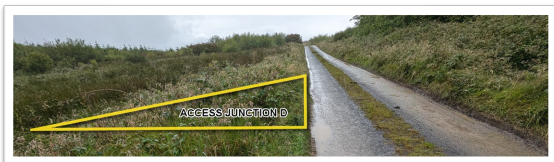
Figure 2.4 – Approach Gradient & Soft Verge Could Lead to Errant Delivery Vehicles Getting Stuck
