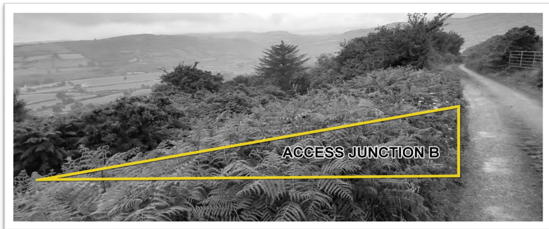
Figure 2.3 – Steep Gradient & Restrictive Horizontal Curvature Could Lead to Vehicle Overturning
